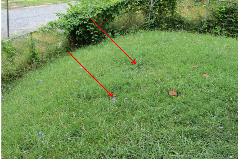
S. 14 th Street – Photo 11 Surface Depressions on Top of Slope in Front of House No. 1426
